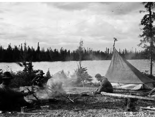
Figure 39—Survey camp near Hudson's Bay height of land (NWT). Library and Archives Canada / PA-020023. 1923
